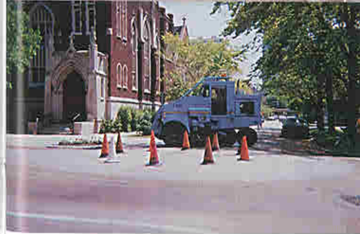
A Chicago Streets and Sanitation vehicle does a trial run around orange cones before the installation of a traffic circle.
