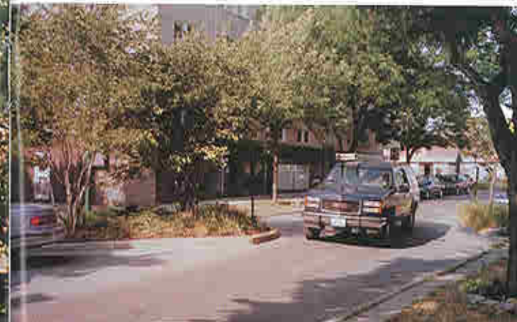
A landscaped chicane slows traffic on a residential street near a school. Chicanes are curb extensions that alternate from one side of the street to the other, grabbing the attention of drivers and forcing them to slow down.
