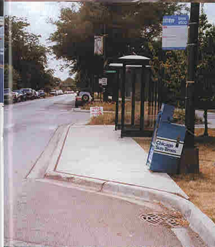
A bus bump-out on Marine Drive prevents traffic from coming up from behind the bus while passengers board. In addition to protecting passengers boarding the bus, it also has the effect of generally slowing traffic on the rest of the street.
